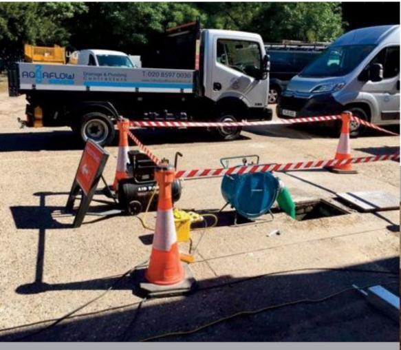
When a pipe becomes broken, cracked, or displaced joints occur, the simplest and most cost-effective way of repair in many cases is to insert a resin based felt liner, or a patch repair, to the pipe.
